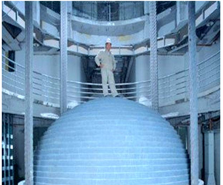
Fig. 3 Tuned mass damper pendulum at Taipei 101.
